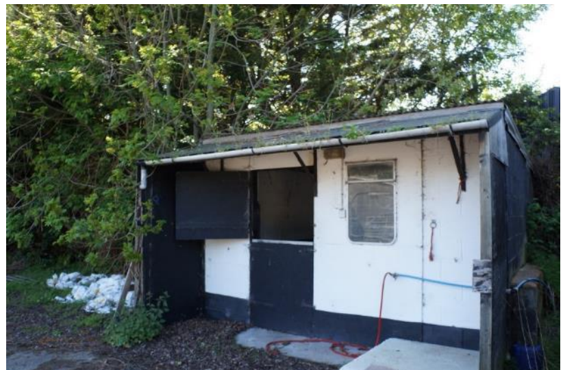
Figure 24: B12: single stable with block and timber walls.
