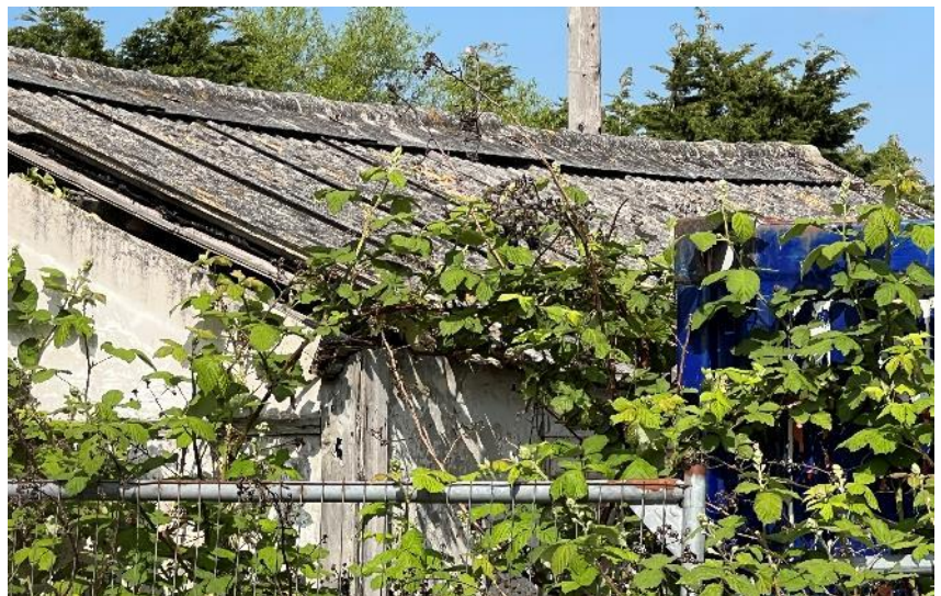
Figure 28: roof materials of B16.
