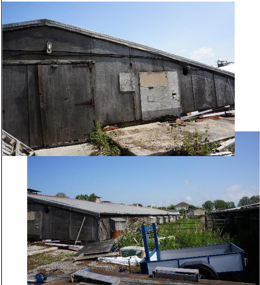
Figure 22: B10 examples of timber poultry sheds on site, in a poor state of repair.
