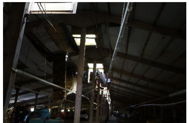
Figure 23: Typical shed interiors with missing sections in both roof and sides.
