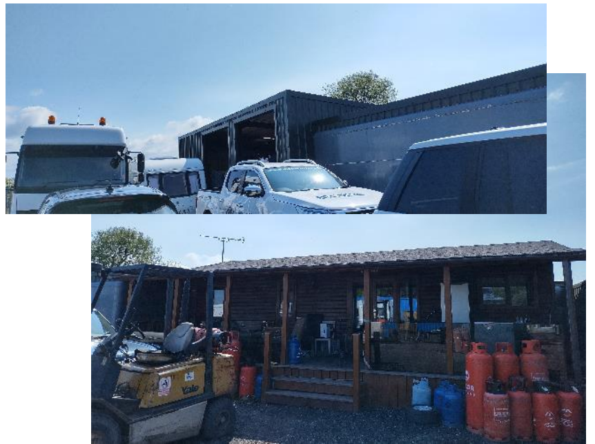
Figure 25: B13: Motor repair garage building.
