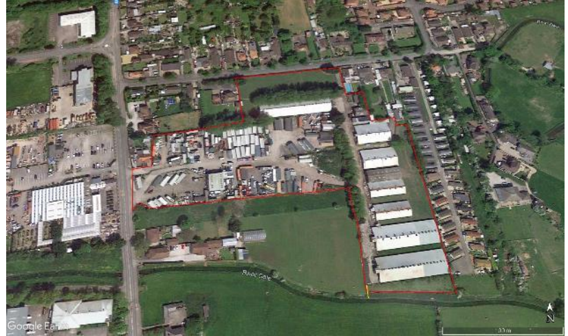
Figure 2: Aerial view of the site ( Google Earth Pro 2023 ).
