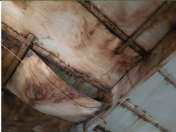
P11: View of the ceiling of the southernmost poultry house.
