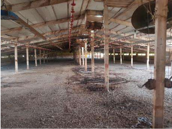
P9: Inside view of the southernmost poultry house with hardstanding floor.
