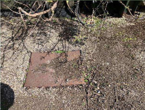
P17: Manhole located in the north-east of the site.
